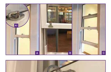
To open your vertical sliding window you need to use the key to unlock the sash lock (A1) then release the catch by turning it 180° you can then use the two sash lifts (B) to open and close the bottom sash in to the required position (C).
