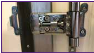
High security hinges anchored into steel reinforcing
