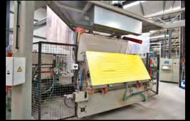
Door manufacturing plant
