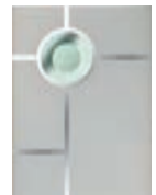
Scotia – clear glass with Zinc and Brass Caming
